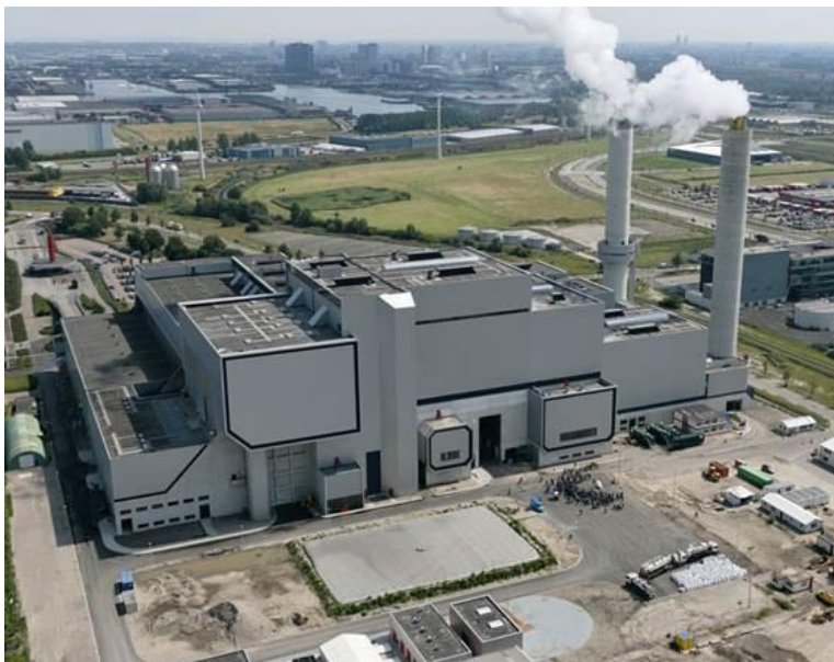
Figure 1-1 AEB waste incineration plant (source: internet/public domain)
